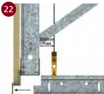
■ VERTICAL SCREW-FIX SYSTEM DETAIL
